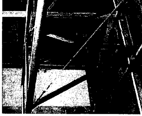
Photo: Installed lift strut and wire bracing.
