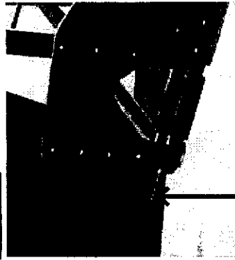
Photo: Gusset plate and five rivets at top of leg
