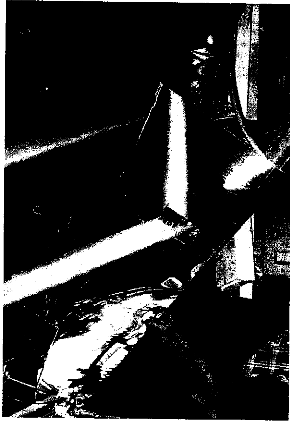
Photo: Attaching the leading edge sheeting.
