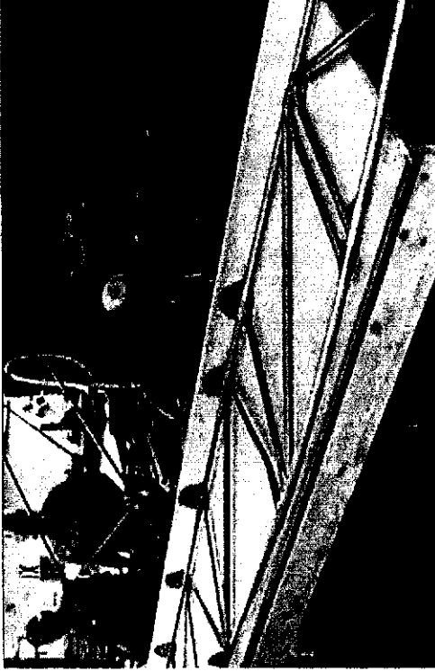
Photo: Round gussets attached and bent.
